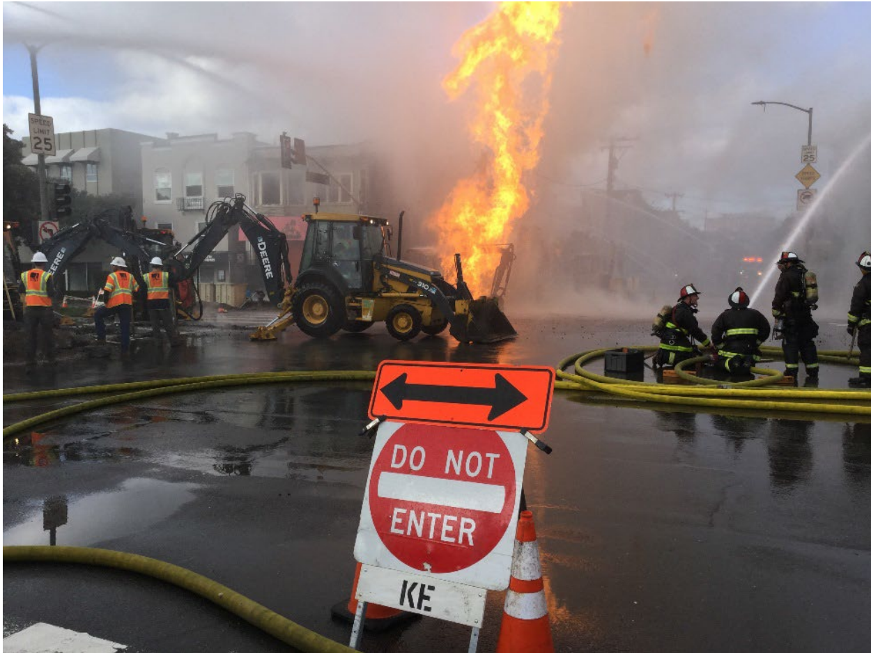
Figure 1. Northwest-facing view of fire during emergency response. (Photo courtesy of PG&E.)
