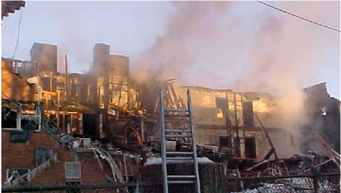
Figure 1. Damage caused by explosion.
