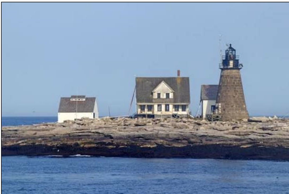
Figure 3. Lighthouse (“watch tower”) on Mount Desert Rock. (Source: Jeremy D’Entremont, newenglandlighthouses.net )
