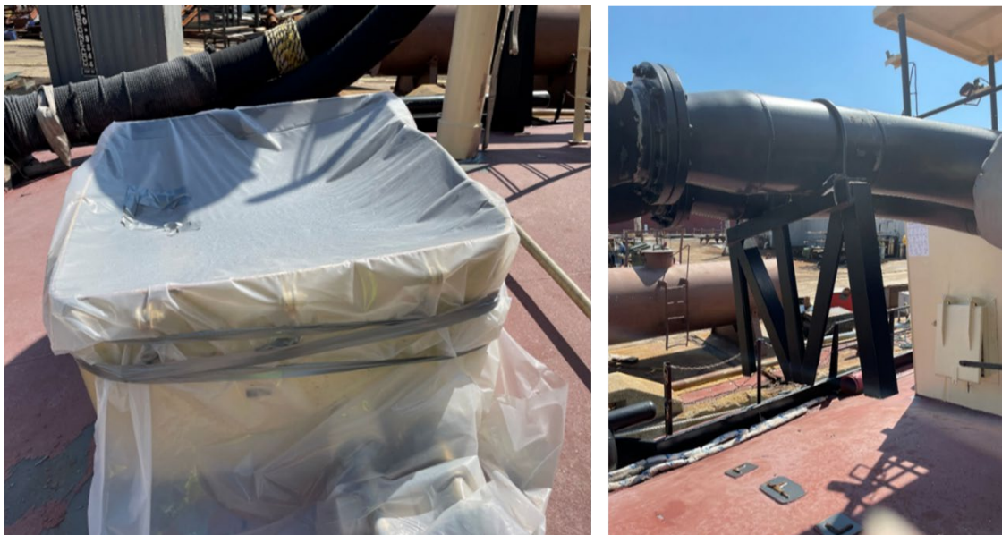
Figure 7. Damage to vessel following the May 24, 2025, explosion. Left to right: Hatch to the no. 2 port cargo tank submersible pump covered in plastic, with hatch cover shown missing. Deformed cargo piping on deck.
