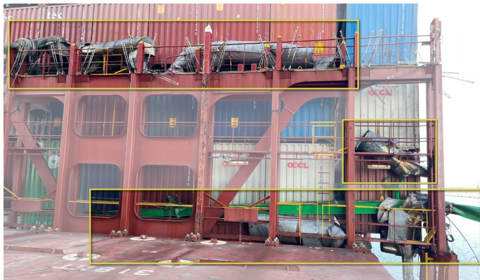
Figure 8. Areas of Erving container bay 83 where sections of the STAX 1 emission capture boom fell (outlined), causing damage.
