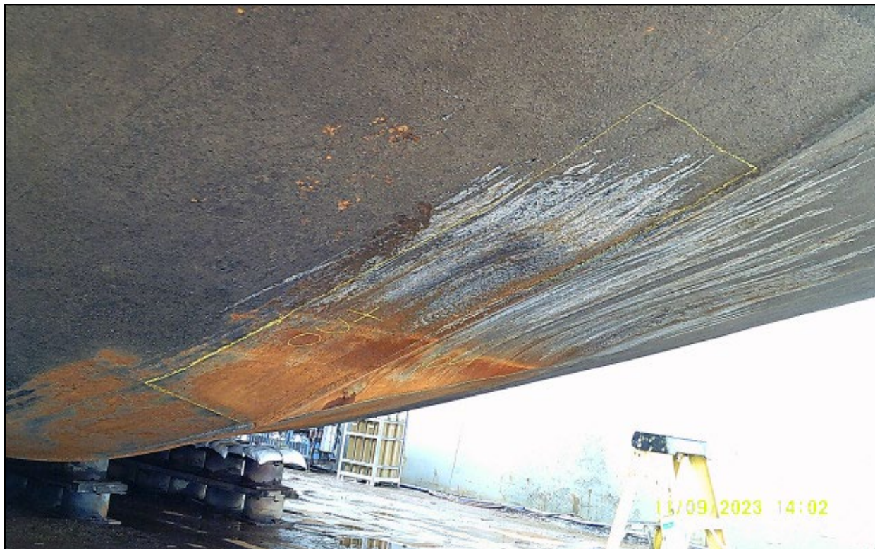
Figure 4. Bottom plating near the bow of the John M Donnelly that was inset when the vessel grounded. (Source: Budwine and Associates, LLC)
