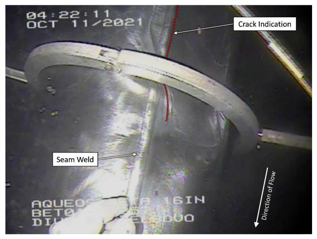
**Figure 6.** San Pedro Bay Pipeline underwater nondestructive testing showing a portion of the crack indication, highlighted in red, on the pipe on October 11, 2021. (Background source: Aqueos)
