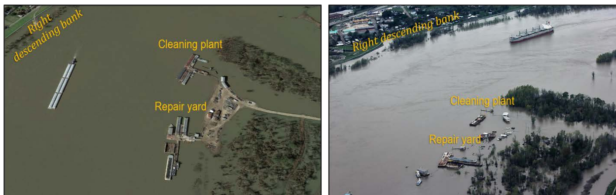
Plaquemine Point Shipyard in January 2019 (left) and immediately after the accident during major flood stage (right). (Source: Google Earth Pro [left]; Coast Guard [right])
