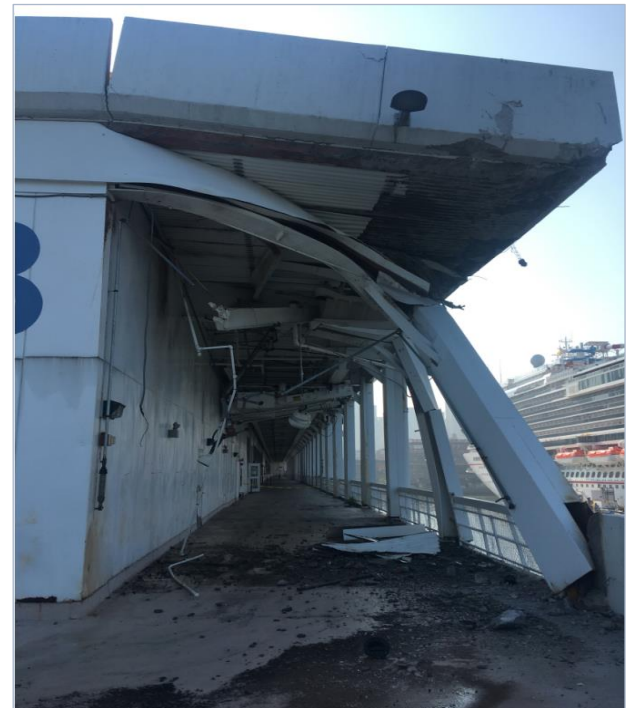
Left, structural damage to Pier 90's parking garage. Right, passenger embarkation walkway among damaged and sagging concrete slabs and metal debris. (Source: US Coast Guard)
