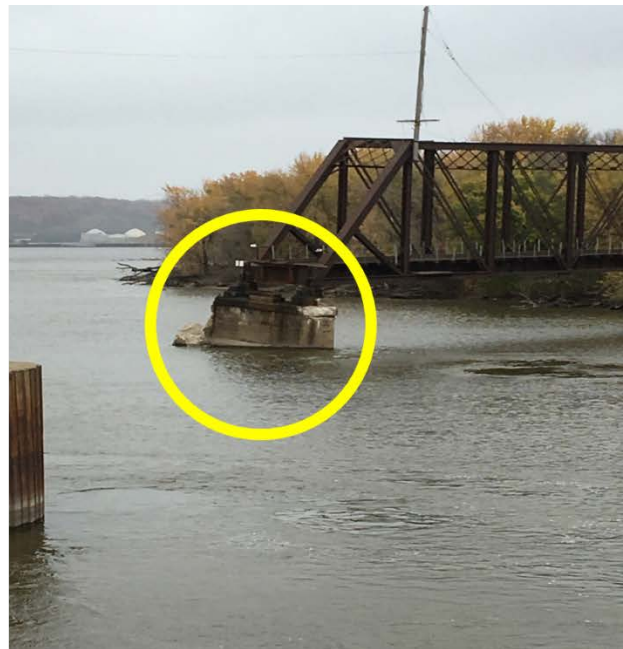
Damage from allision: (at left) raked bow of port lead barge, ART 35157 ; (at right) fixed pier of swing bridge near left descending bank struck by barge (downstream view).
