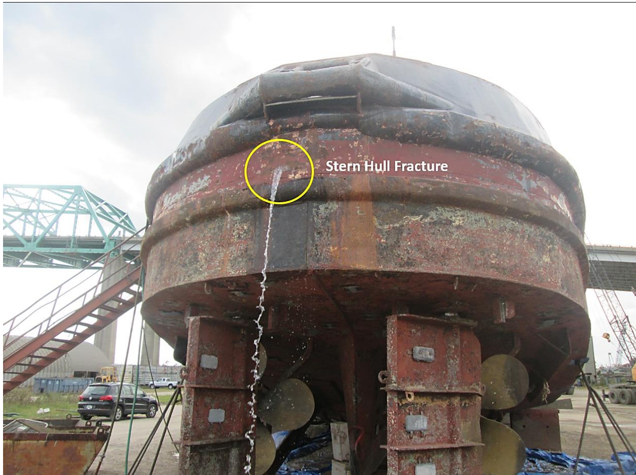
Stern hull fracture discovered in drydock. (Photo with permission of A. P. Boudreaux, surveyor)
