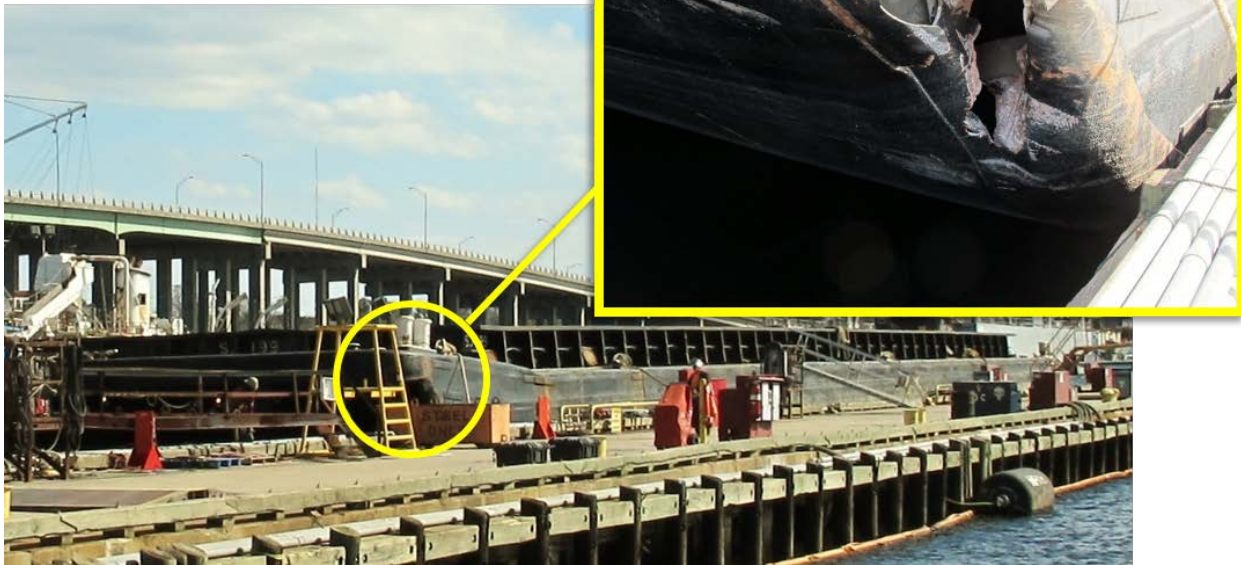
Barge SJ-199 docked at the repair yard.
