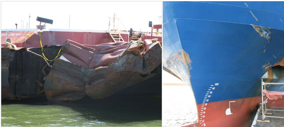
At left, damage to the starboard bow of the Kirby 28044 . At right, damage to the port bow of the Ocean Freedom .
