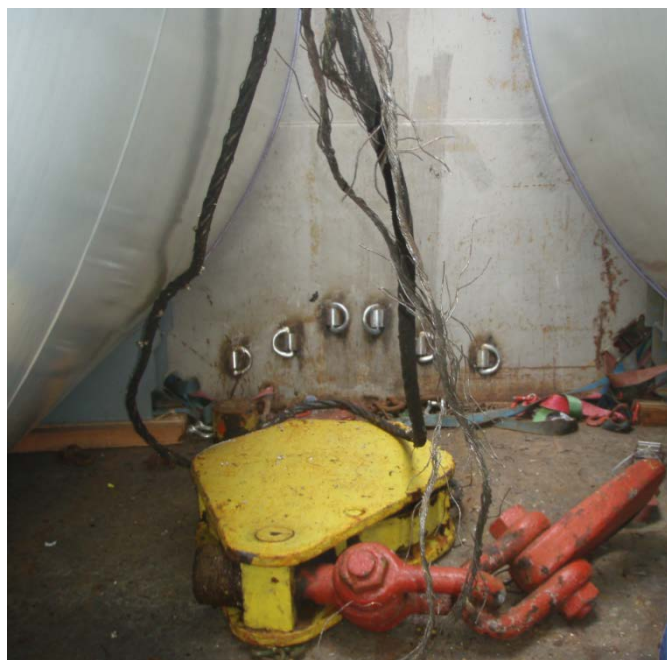
Lifting block, with hook and broken wire rope, for crane no. 4 that fell to the bottom of cargo hold no. 4.
