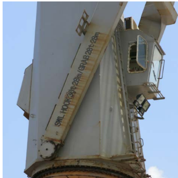
Crane no. 4 with its jib left in position after the cargo was dropped.
