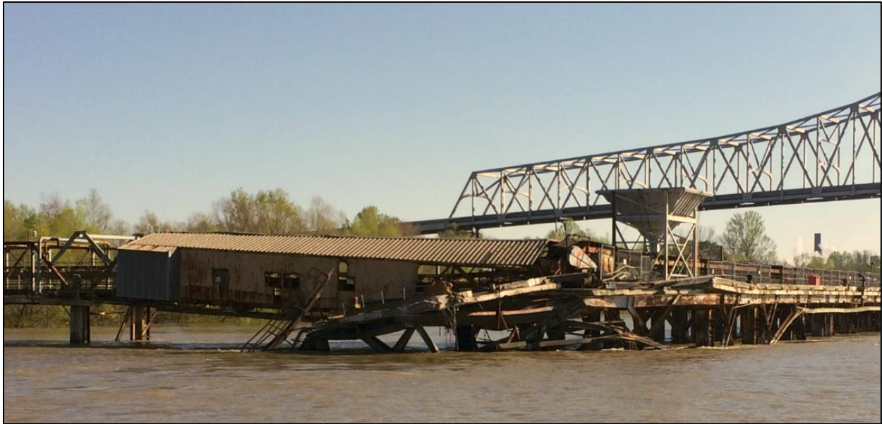
Damaged LSR raw sugar unloading dock. (Photo by Coast Guard)
