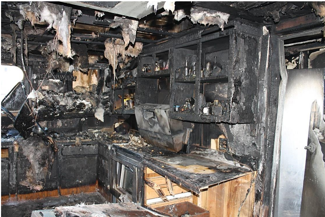
Fire damage to the San Gabriel galley located on the main deck. (Photo by Coast Guard)
