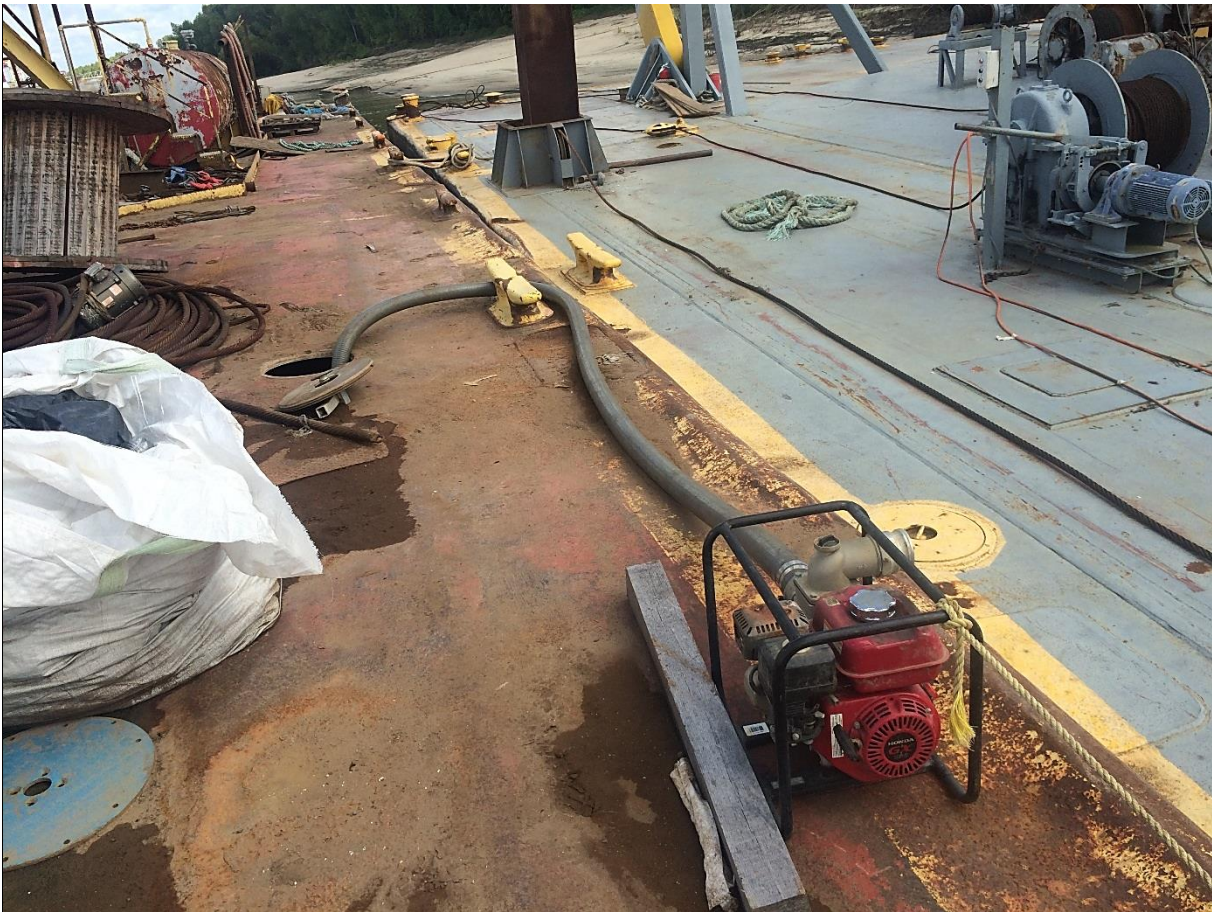
Portable pump and hose rigged to dewater a void on deck barge Bulk Crane 3 .
