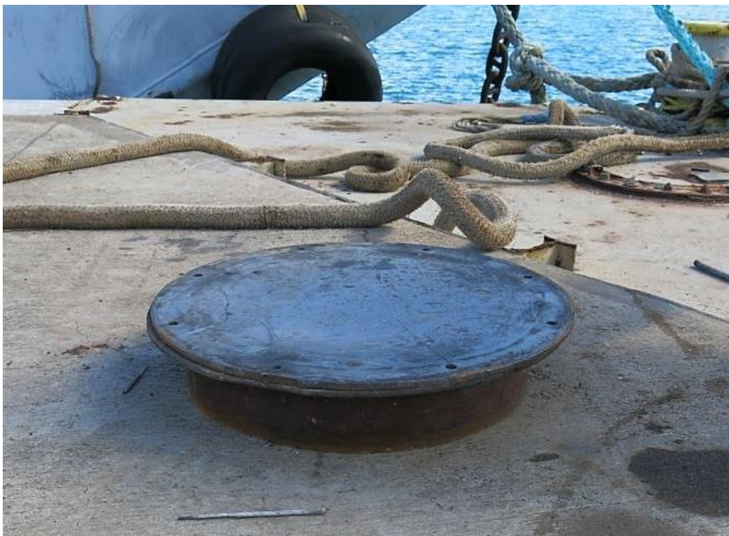
The replacement cover that was to be installed on the starboard aft peak tank.
