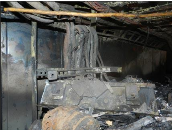
Damaged electrical cables and cable tray, left, and motor control center, right. (Photos courtesy Oceaneering International)
