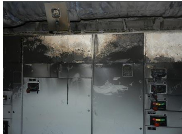
Damaged electrical cables and cable tray, left, and motor control center, right. (Photos courtesy Oceaneering International)
