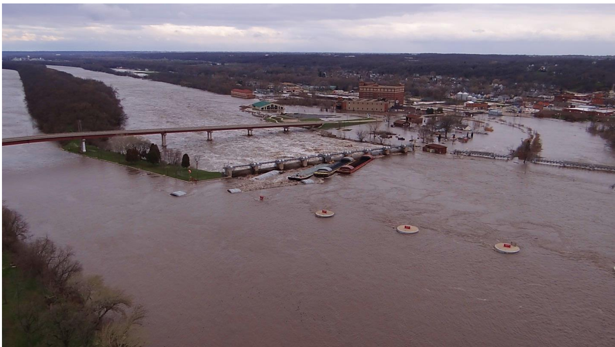
The Marseilles Dam after the barges broke away. Several barges can be seen pushing against the dam. The city of Marseilles, seen in the top right of the photo, flooded. (Photo by the Coast Guard)
