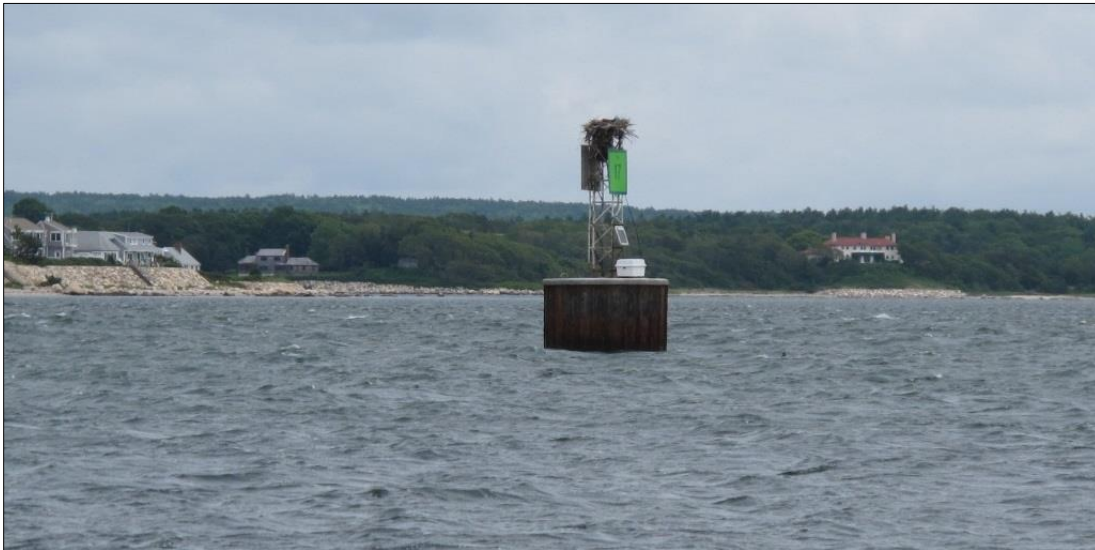
Looking east at light 17 in Hog Island Channel. The structure is 24 feet high and flashes a green light every 6 seconds.
