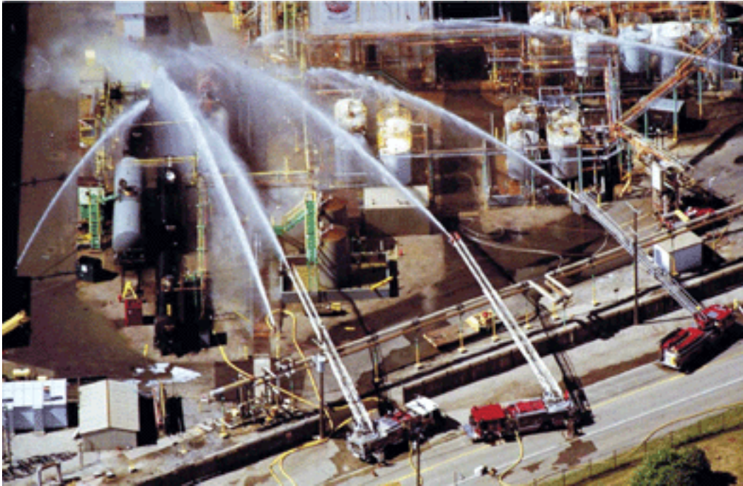
Figure 3. Overview of accident site and emergency response.
