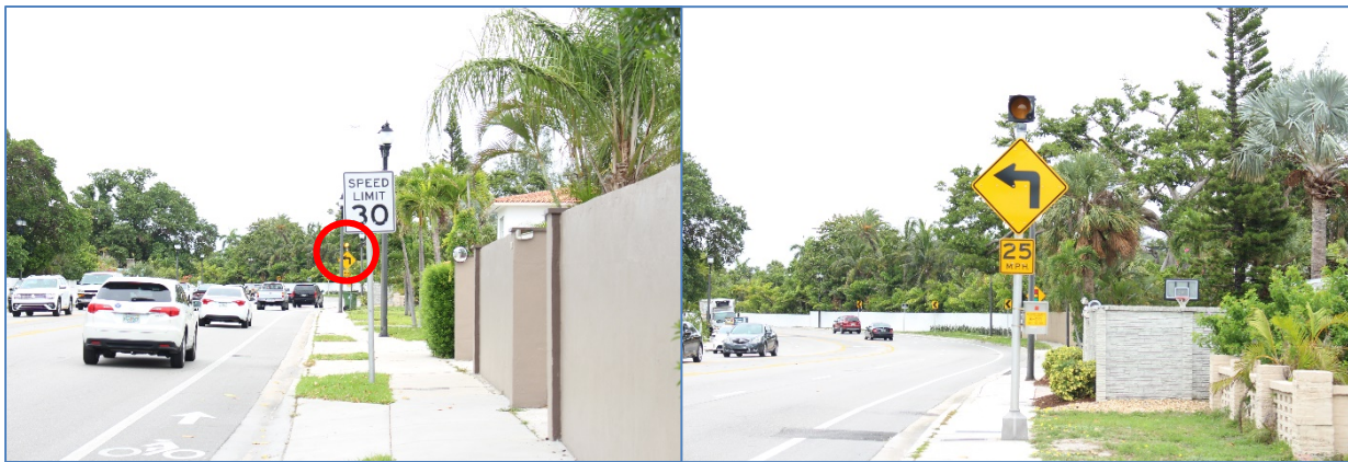
Figure 1. Seabreeze Boulevard with advance warning sign circled in red; and closeup view of approach to curve with advance warning sign, flashing beacon, and 25-mph advisory speed limit.
