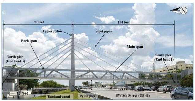
pier, across the Tamiami Canal, and end at the north pier at the same height elevation (see figure 2).<sup>1</sup>
