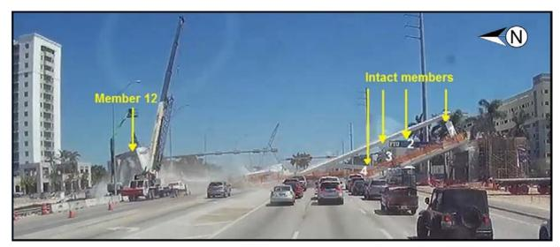
**Figure 11.** Still image (time stamp 13:46:44:310) from in-vehicle mounted video camera on pickup truck traveling east on SW 8th Street, showing main span completely collapsed, March 15, about 1:46 p.m.
