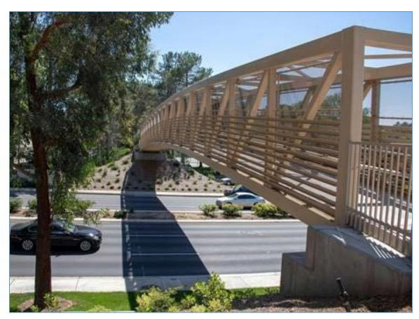
Figure 8. Typical truss bridge with one set of regularly spaced vertical truss pieces running along each side, with top lateral bracing constructed of steel. (Source: Santa Clarita, California)
