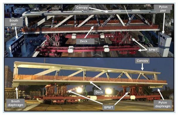
**Figure 22.** SPMT being moved overnight on March 10 (bottom) and main span being placed on south and pylon piers, facing west (top). Transport occurred over 8 hours, starting at 4:30 a.m., with placement of final permanent pier support concluding at 12:30 p.m. (Source: FIGG, annotated by NTSB)
