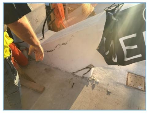
Figure 25. Cracks at bottom of diagonal member 11 (west view), March 15. (Source: FIGG)
