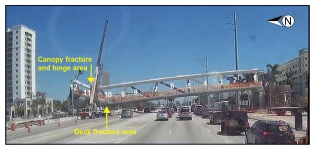
**Figure 10.** Still image (time stamp 13:46:44:046) from in-vehicle mounted video camera on pickup truck traveling east on SW 8th Street, showing full-width canopy fracture and deck fracture areas at north end (pylon pier), March 15, about 1:46 p.m.
