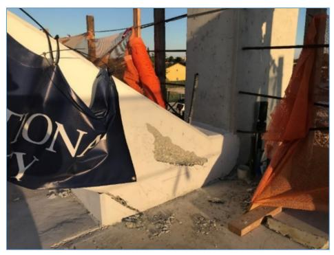
Figure 26. Cracks at bottom of diagonal member 11 (east view), March 15. (Source: FIGG)
