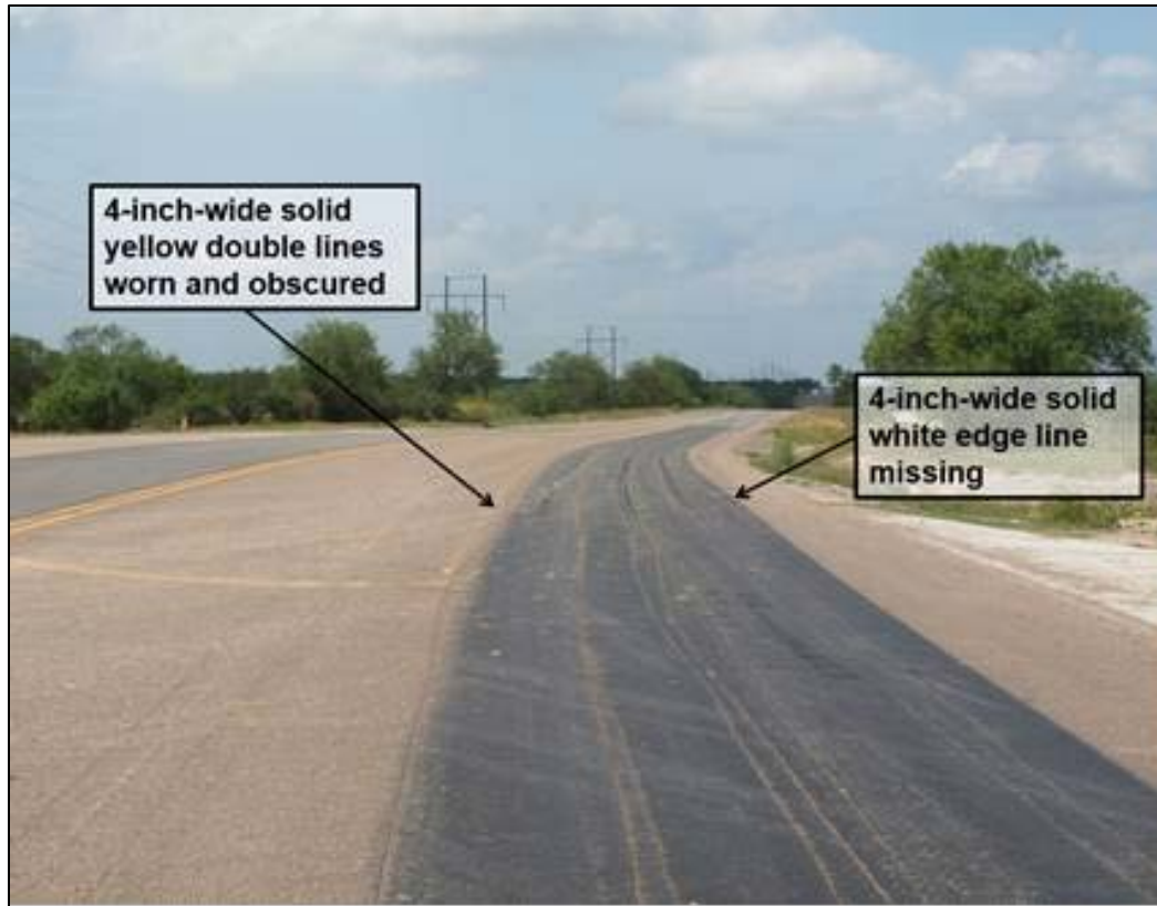
Figure 9. Northbound view of US-83, showing the degraded condition of lane striping within the curve.
