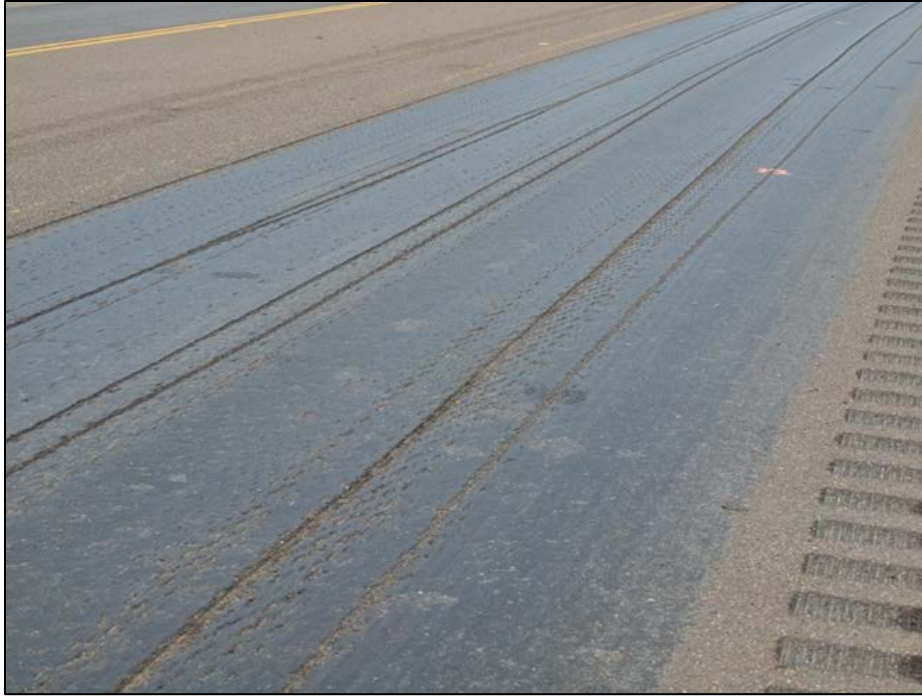
Figure 13. View of US-83 northbound travel lane shortly after the crash, showing gouges and continuous longitudinal grooves in the pavement surface.
