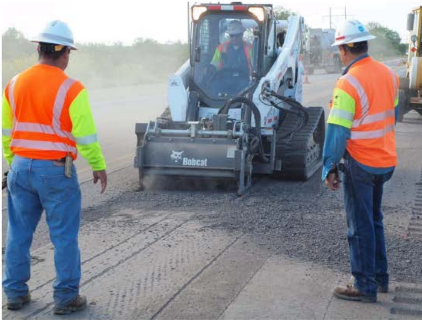
Figure 13: May 18, 2016 milling operations
