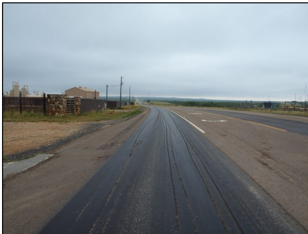
Figure 14. Views of the northbound US-83 lane looking south. The photo on the left shows the northbound travel lane as it appeared in May 2016. The photo on the right shows the northbound travel lane as it appeared in August 2016, after the completion of the successful chip seal operation.
