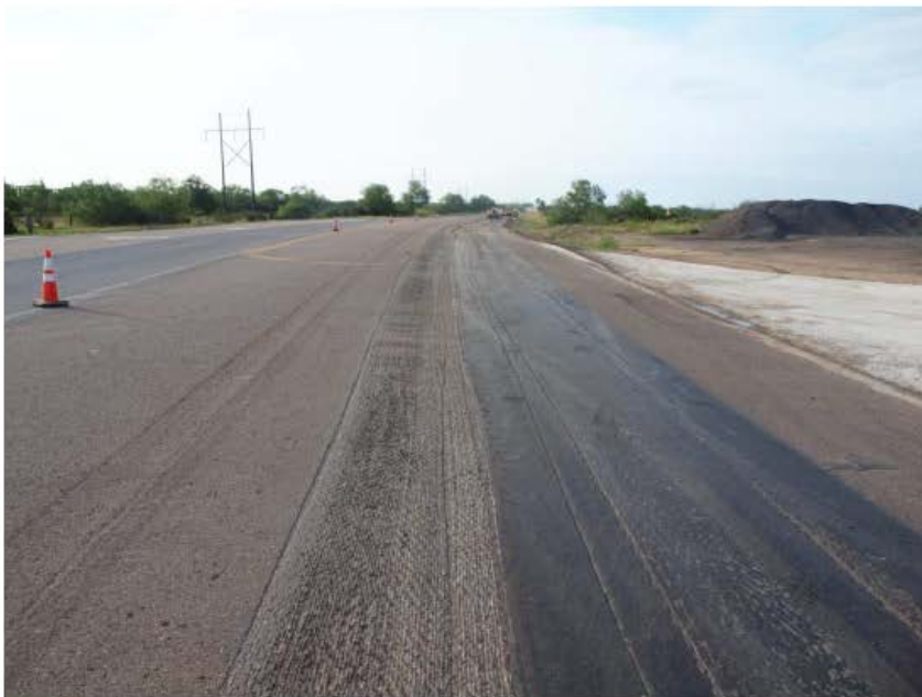
Figure 14: May 18, 2016 milling operations. Note the contrast of the May 18, 2016 milling results (texture) on the left compared to the results of the milling performed on October 26, 2015 on right.
