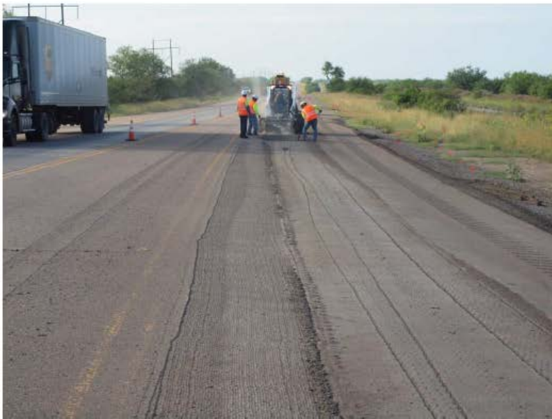
Figure 12: US83 Northbound, looking north from approximately the crest of the vertical curve. TxDOT maintenance forces performing milling on May 18, 2016 using Bobcat-mounted milling drum to restore pavement macrotexture. First pass of the milling drum adjacent to yellow stripe.
