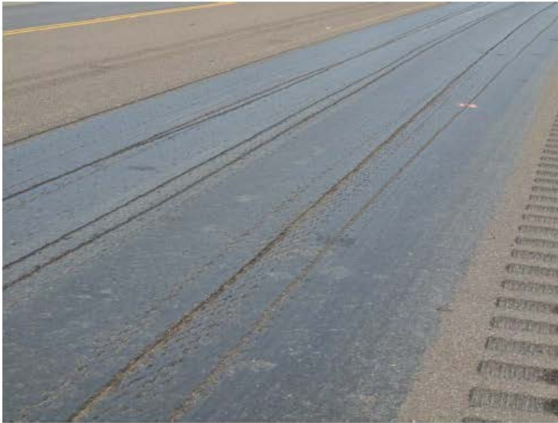
Figure 7: US83 northbound lane, close up of milled section in vicinity of driveways. The longitudinal grooves were reported to be from milling operation. Image obtained by NTSB on 05/15/2016.
