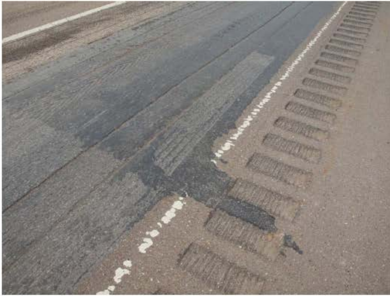
Figure 11: US83 northbound lane, close up of south end of milled section. Note the rumble strip (constructed February 10, 2016) intersects the surface asphalt material. Image obtained by NTSB on 05/18/2016
