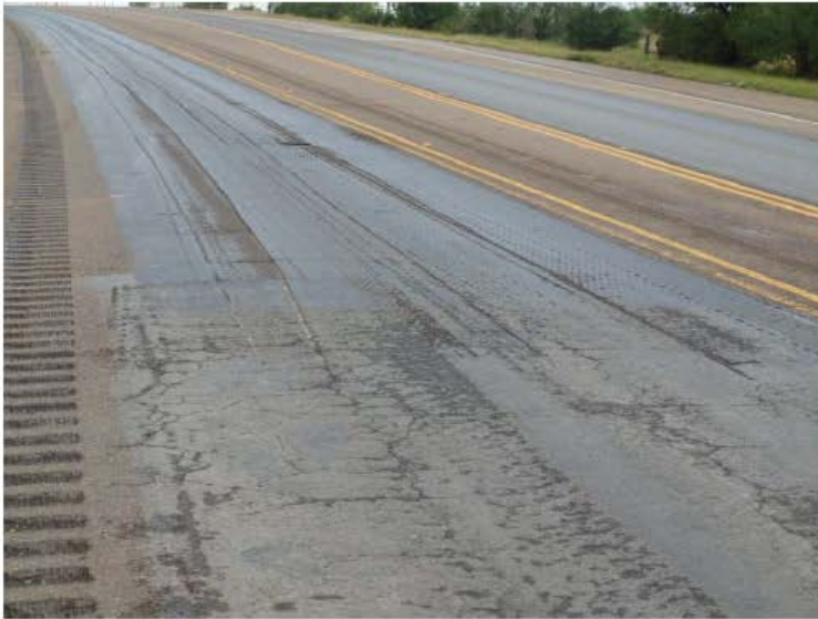
Figure 9: US83 northbound lane, looking south, at end of milled pavement. Note the pavement cracking in foreground is consistent with pavement conditions at time of milling. Image obtained by NTSB on 05/15/2016.
