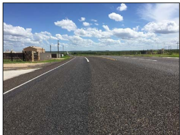
Figure 14. Views of the northbound US-83 lane looking south. The photo on the left shows the northbound travel lane as it appeared in May 2016. The photo on the right shows the northbound travel lane as it appeared in August 2016, after the completion of the successful chip seal operation.
