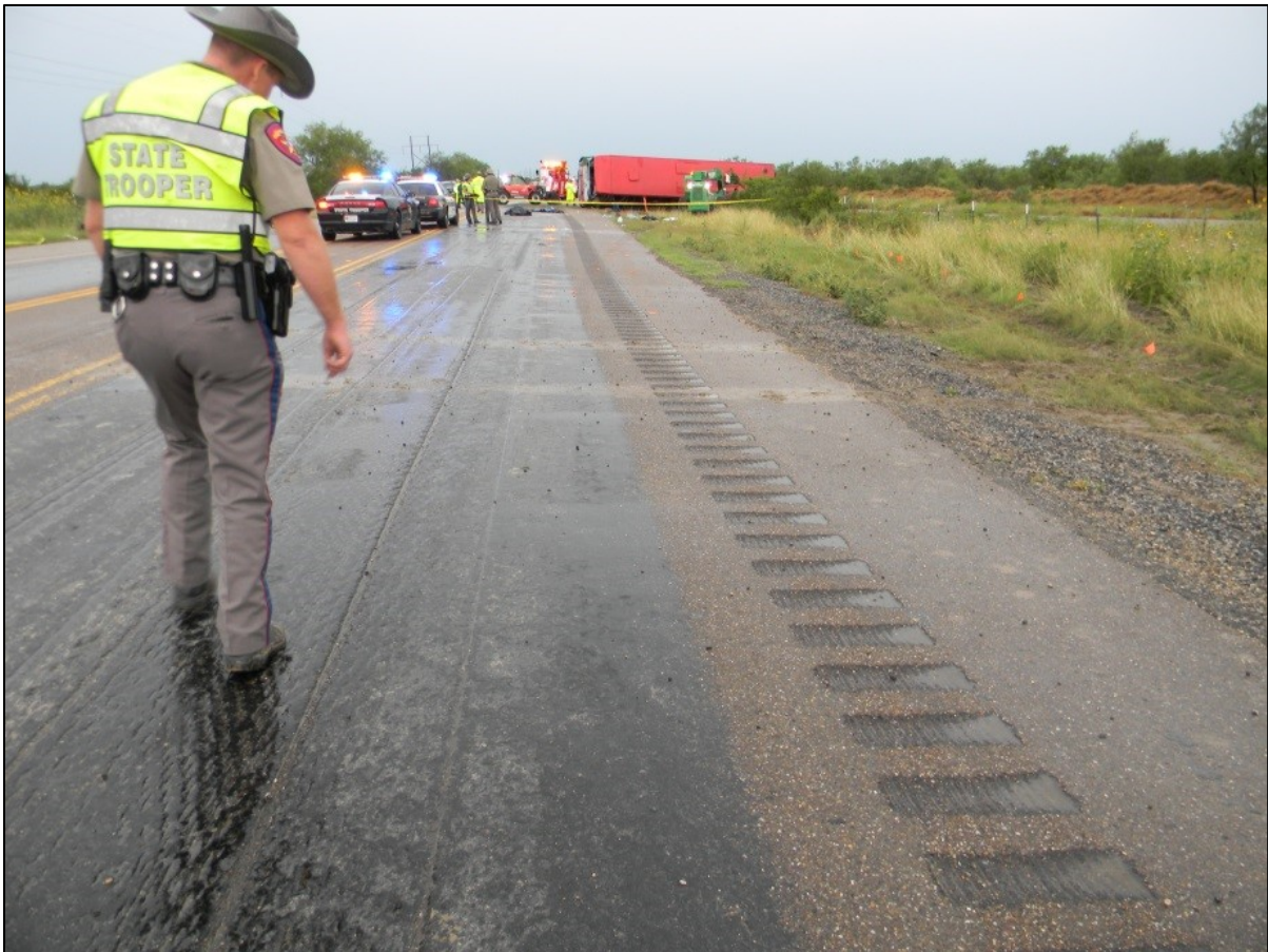
Figure 12. Postcrash view of US-83 northbound travel lane. The slick-appearing surface and increased reflectivity contrasts with the paved shoulder on the right. (Source: TxDPS)
