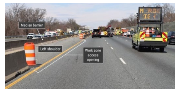
FIGURE 18. Postcrash view of the work zone and the opening in the concrete barriers through which the Acura entered.
