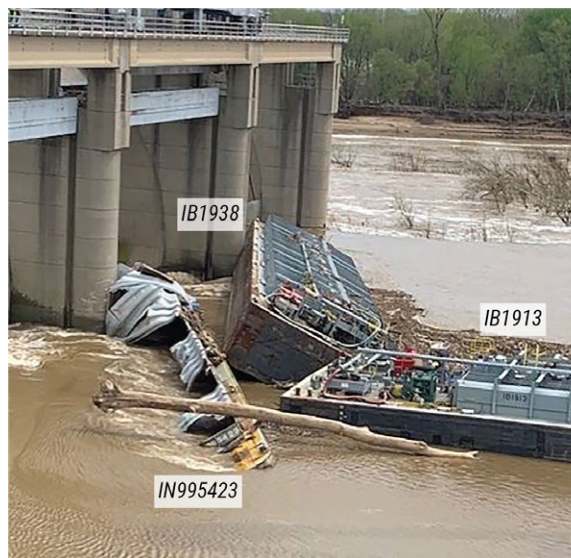
FIGURE 30. Barges IN995423 and IB1938 against the lower dam gates. IB1913 is receiving methanol from IB1938 through a cargo transfer hose.
