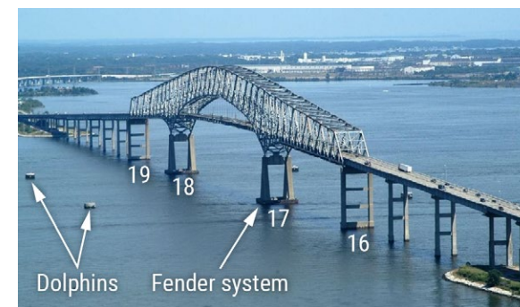
FIGURE 15. The Francis Scott Key Bridge in 2004 showing piers 16 through 19 and the physical features—dolphins and fendering system—designed to protect the bridge from vessel traffic.
