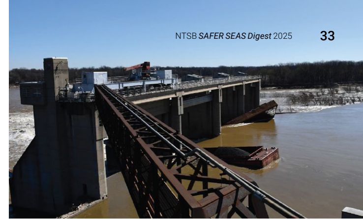
Barges from the Amber Brittany tow lodged in the Lower McAlpine Dam Gate after the tow broke apart.
