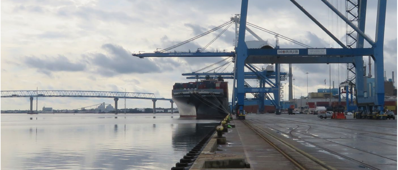
Mooring configuration at North Charleston Terminal similar to the Celsius Nicosia's when the crane on the Royal Engineer tow contacted the STS crane. (The beam of the vessel shown is 25 feet wider than the Celsius Nicosia.).
