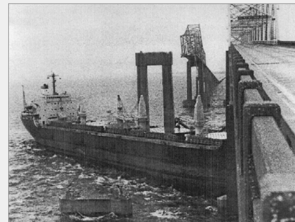
View of the collapsed western span of the Sunshine Skyway Bridge in Tampa Bay, Florida, after the Liberian-flagged bulk carrier Summit Venture rammed a support pier on May 9, 1980. The NTSB investigated the accident and issued recommendations to FHWA and the Coast Guard that ultimately resulted in AASHTO's adoption of its 1991 Guide Specification and Commentary for Vessel Collision Design of Highway Bridges , which introduced a vulnerability assessment calculation for bridges.
