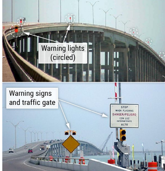
Safety features installed on the rebuilt Queen Isabella Causeway (now known as the Queen Isabella Memorial Bridge). BACKGROUND SOURCE: TXDOT.
