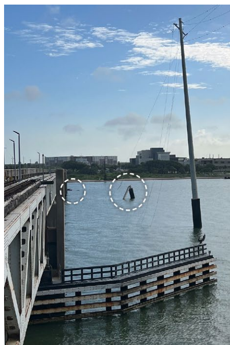
The damaged power transmission poles, in the foreground and circled with a dotted line. The smaller circle indicates the debris/damage to one of the bridge's piling clusters, seen right. SOURCE: COAST GUARD.
