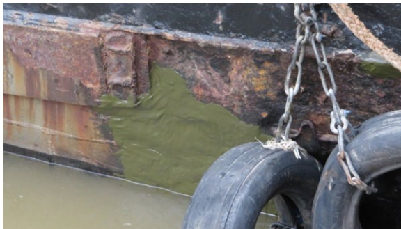
Temporary epoxy repair, applied during the postcasualty salvage, on the port quarter, near the lazarette.
