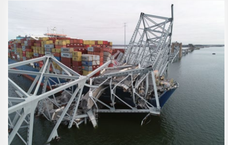
ON THE COVER: The containership Dali with portions of the collapsed Key Bridge across its bow (page 46).
