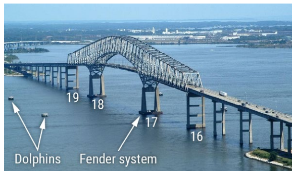
The Francis Scott Key Bridge in 2004 and the physical protection systems (dolphins and the pier fendering system) protecting piers from vessels transiting under the Key Bridge.
