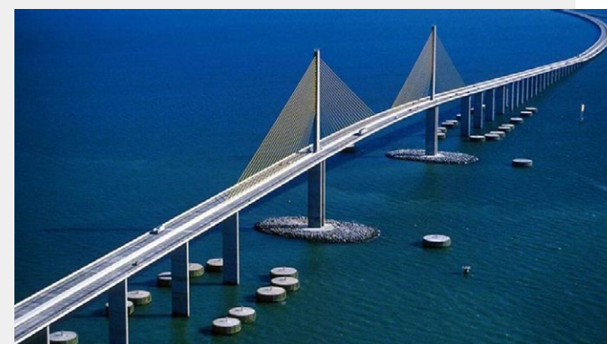
The rebuilt Sunshine Skyway Bridge showing the dolphin and island protection system.
