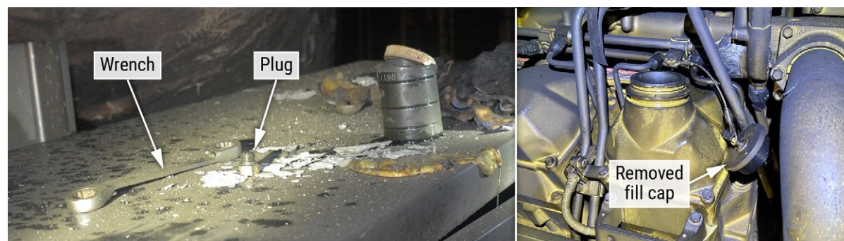
Removed plug on top of a storage cabinet and the removed fill cap from the port auxiliary engine.
