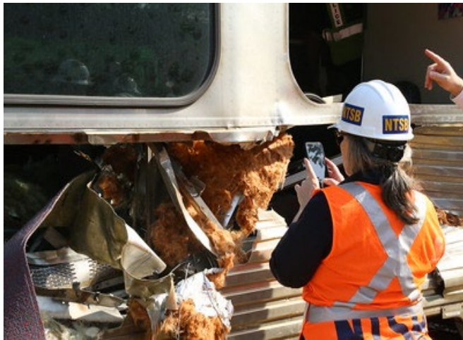
Figure 6. NTSB investigator documenting damage to the train involved in the grade crossing collision between a Metra train and truck near Clarendon Hills, Illinois.
