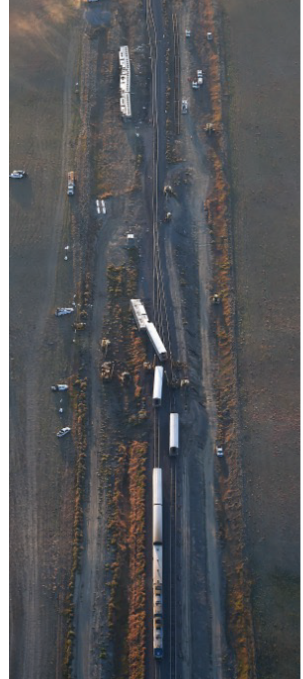
Figure 30. Aerial view of the Amtrak train derailment with passenger fatalities near Joplin, Montana, September 25, 2021.
