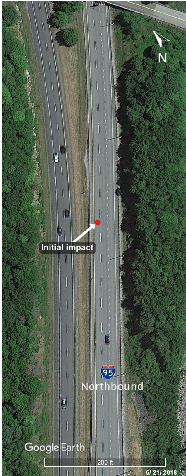
Figure 2. Overhead view of the crash site, showing the three northbound lanes of I-95 on the right. (Source: Google Earth modified)
