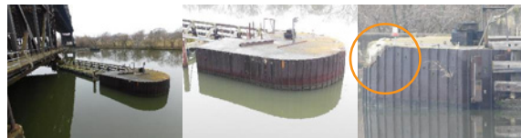
Figure 121. Left and center: Northeast protection cell for Rock Island Railroad Bridge. Right: View from across the river of damaged protection cell with impact location circled. SOURCE: CSX TRANSPORTATION.
