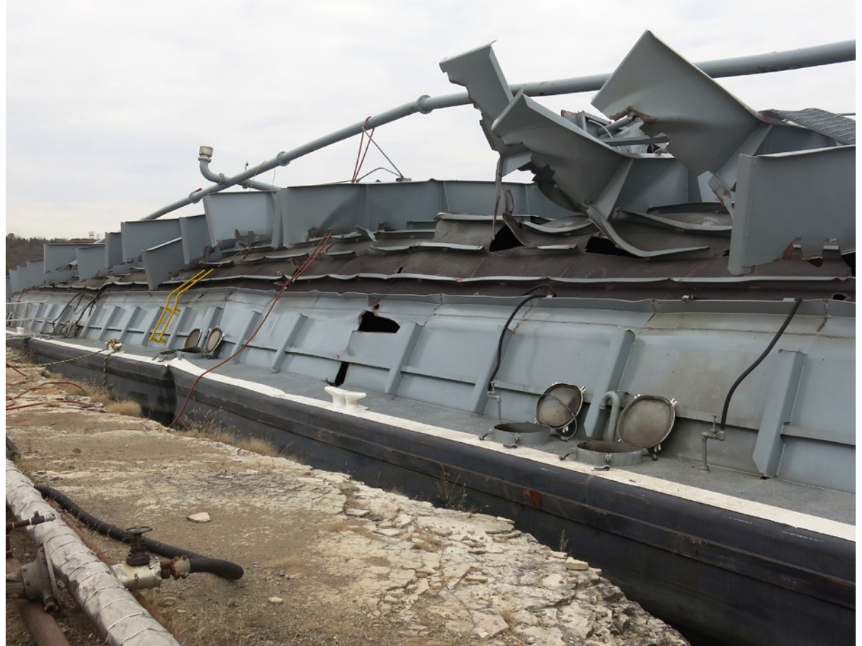
Figure 150. Damage of the IB1940 after the explosion shows a distorted portside tank bulkhead and raised tank-top.
