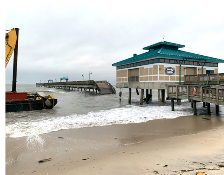
Figure 124. The damaged fishing pier with debris on the deck of the YD 71 .
