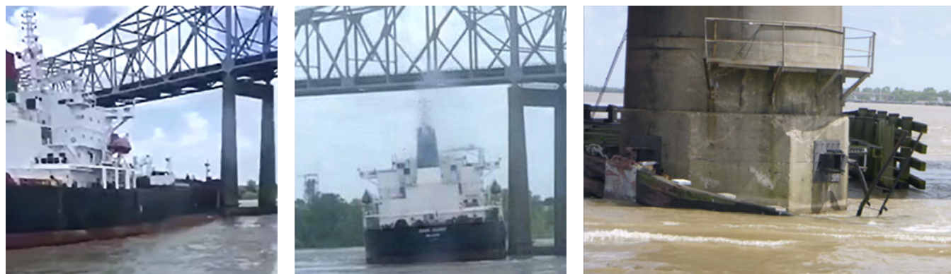
Figure 65. Left and middle: Two photos showing the Dank Silver striking the Sunshine Bridge. SOURCE: CRESCENT TOWING. Right: Damage to the fendering system for the western pier of the Sunshine Bridge, from the north. SOURCE: LOUISIANA DEPARTMENT OF TRANSPORTATION AND DEVELOPMENT.
