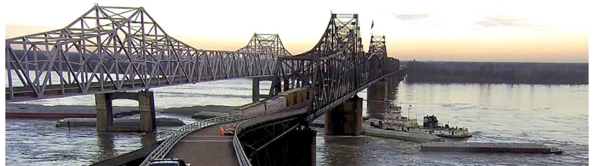
Figure 59. Barges broke away from the Chad Pregracke after the tow struck pier 3 of the Old Highway 80 bridge.
