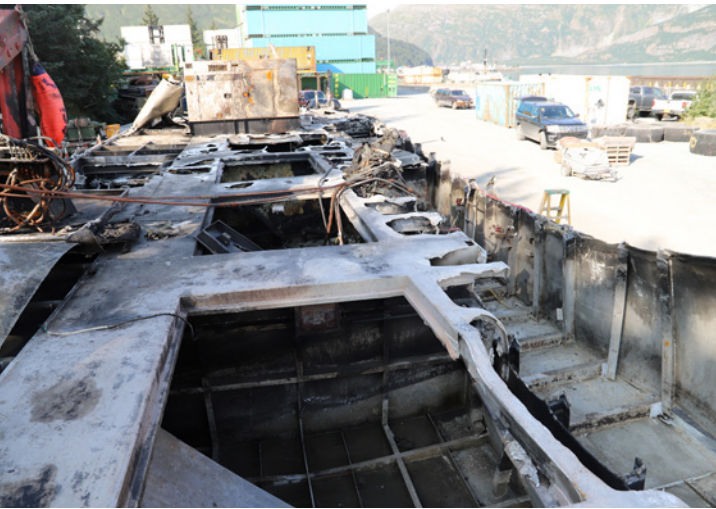
Figure 127. Bent and deformed deck plating forward on the Alaganik 's starboard pontoon after the fire.
