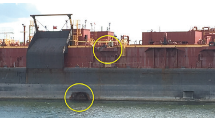
Figure 39. Damage to OSG 243 , port side. Yellow circles identify, at top, cantilever deck damaged by Yochow 's bow rake and, at bottom, side shell at waterline in no. 5P ballast tank penetrated by bulk carrier's bulbous bow.
