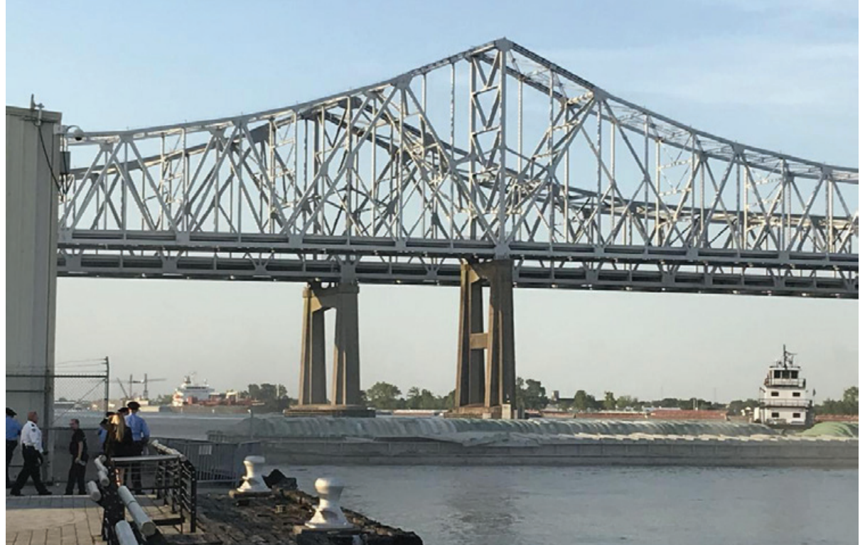
Figure 69. Steve Richoux and barges after the accident (view downriver with the Crescent City Connection Bridges in the background). SOURCE: MARDI GRAS WORLD
