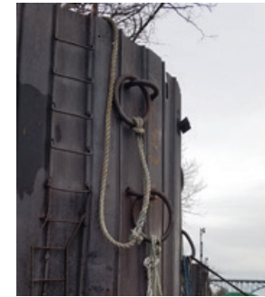
Figure 50. A piling at Jacks Run with mooring rings as designed.
