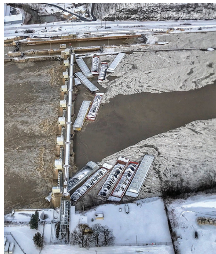
Figure 48. Aerial photo of Emsworth Locks and Dam with breakaway barges. SOURCE: COAST GUARD
