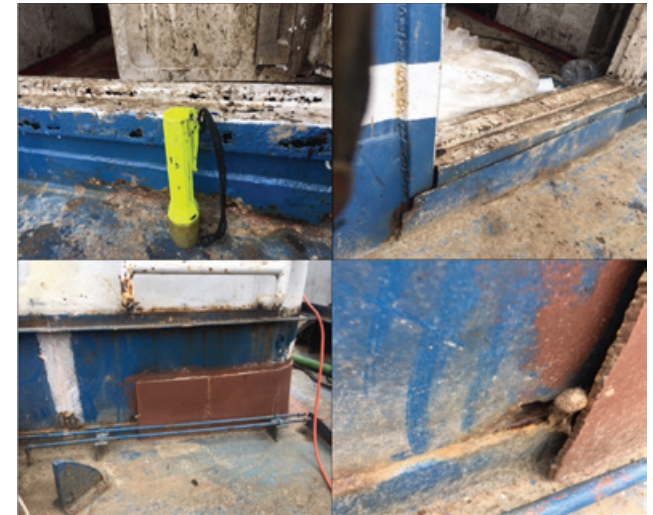
Figure 131. Wastage and doubler plates as found on Ms Nancy C deckhouse. Top left: doubler plate over wastage below starboard engine room entrance. Top right: doubler plate over wastage below port engine room entrance. Bottom left: doubler plates over wastage on starboard aft deckhouse. Bottom right: close-up of starboard aft doubler plate showing gap between plate and wastage area.
