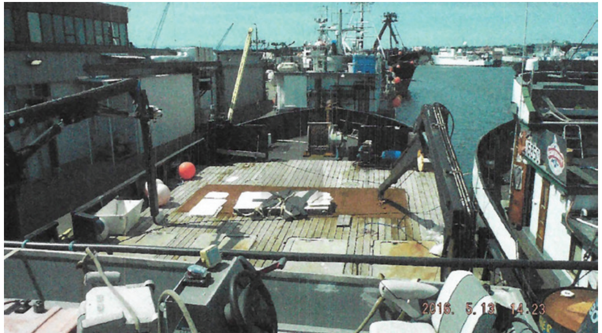
Figure 112. Photo from a 2016 survey report documenting the condition of Logger shows wooden deck boards on the main deck, from where the captain saw smoke emanating.
