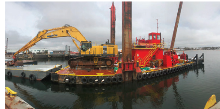
Figure 6. Dredge200 with excavator boom extended.
