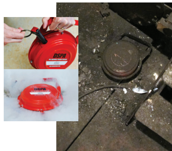
Figure 122. Below: grenade-type aerosol fire extinguisher used initially to combat the fire sits on the deck of the engine room near the entrance ladder. Inset: two photos from the manufacturer's website demonstrate how the device activates.
