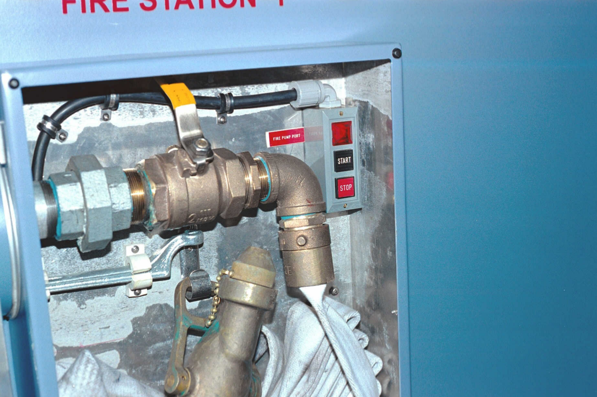
Photo - fire station
