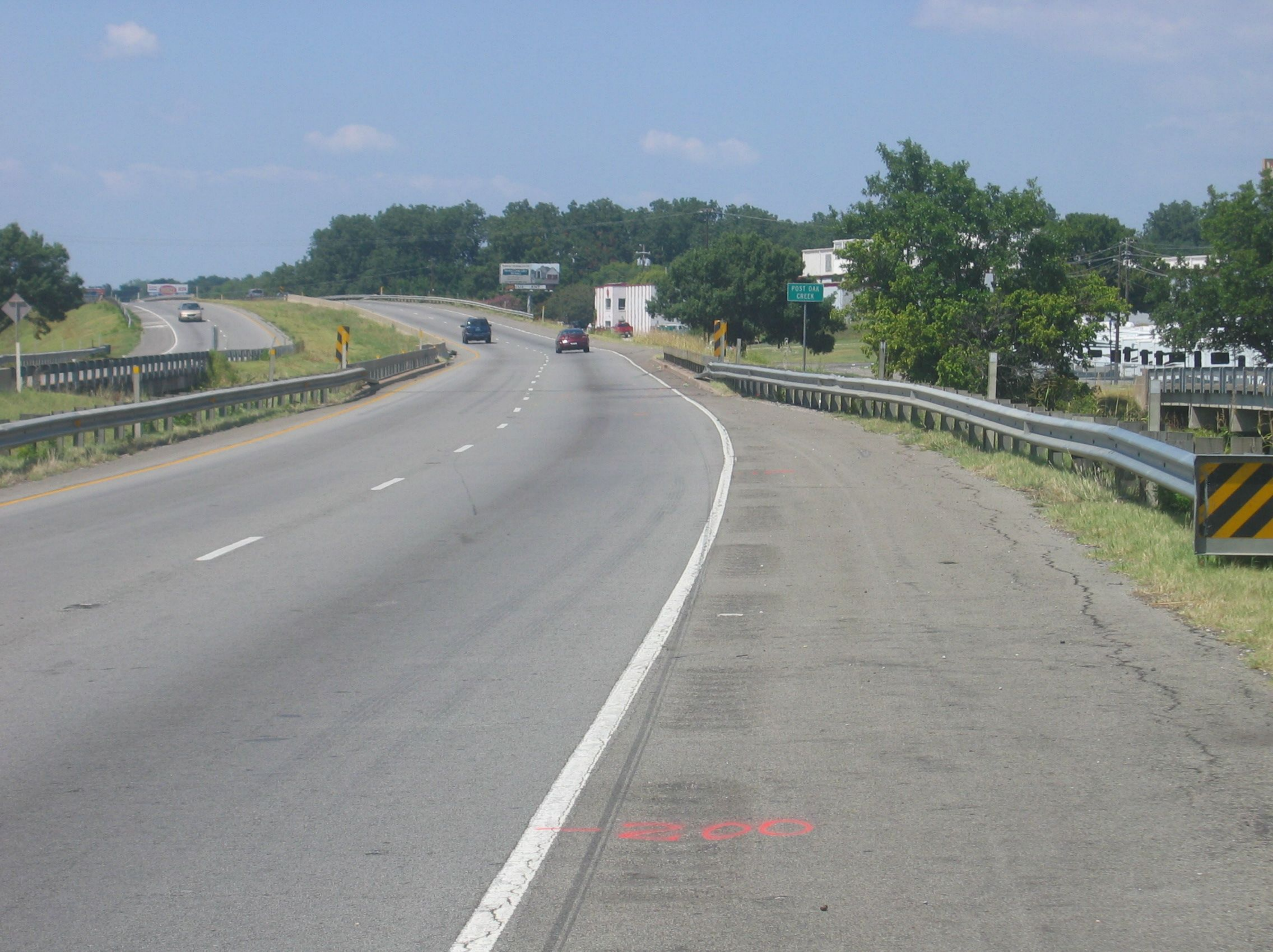
HWY PHOTO 10, View of Approach to Postoak Creek Bridge from Approximately 200 feet.
