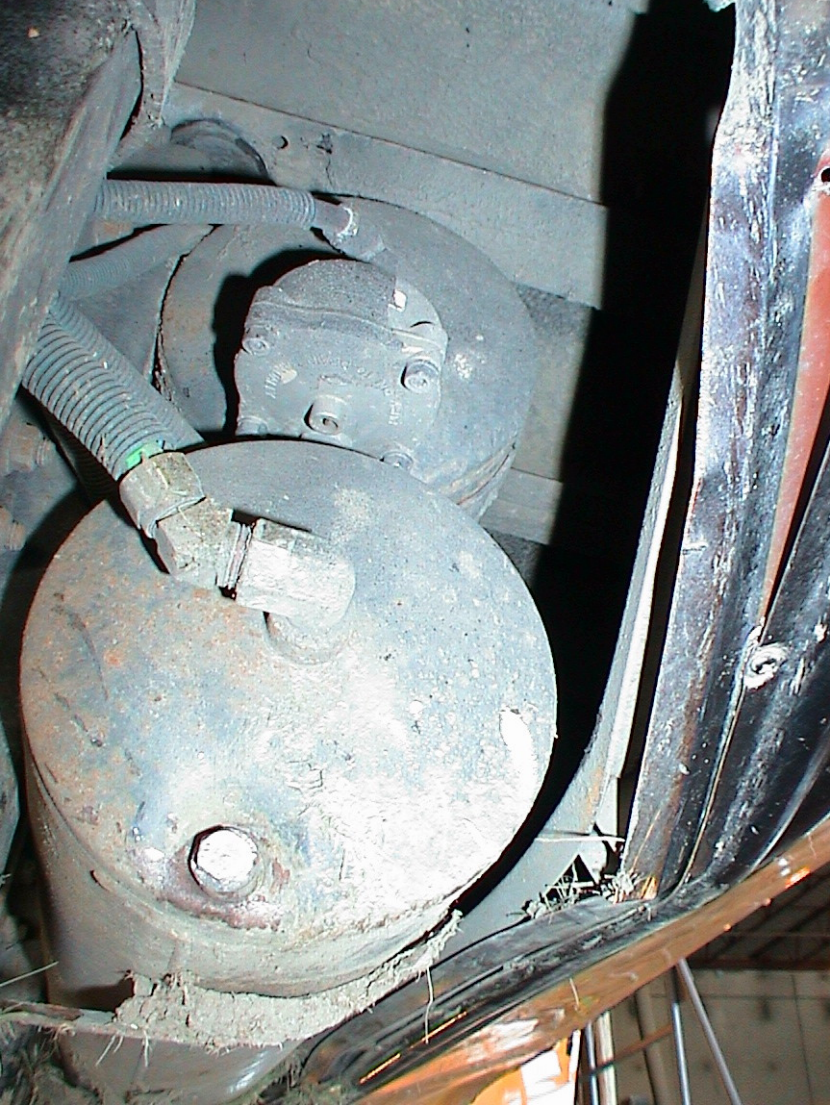
VEH Photo #15 - Left Front Air Tanks Showing Plug Where DV-2 Valve Was Broken Off
